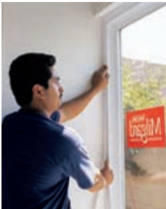
STEP 3: INSULATE AND TRIM Perimeter insulation is added to seal drafts, and interior trim, which varies by dealer, to create a finished look.
