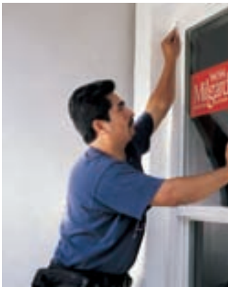
STEP 2: REMOVE OLD UNIT, INSTALL NEW WINDOW Your Milgard dealer is experienced with which method of installation is best for each type of exterior finish.
