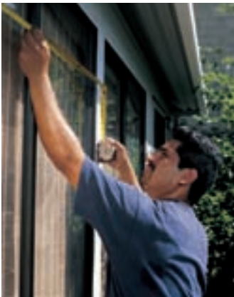
STEP 1: MEASURE OPENING Before any window or door is removed, the openings are carefully measured to make sure every unit is built to your required size.
