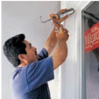
STEP 4: SEAL AND FINISH EXTERIOR Seal to make watertight and touch-up. That's it.
